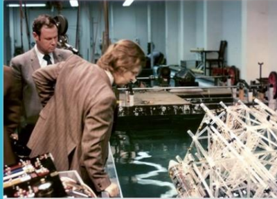
Before computers could simulate installation scale models were built
