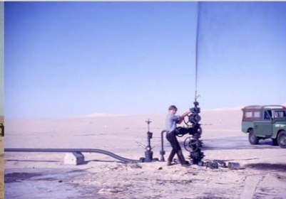
Bleeding tubing prior to dead-weight testing, Libya 1966
